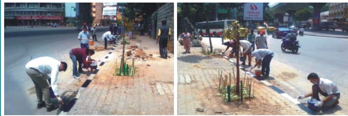
Relaying the broken cobble stones & painting the footpath
